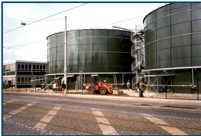
BECKs pretreatment facilities operated by hansewasser Bremen
