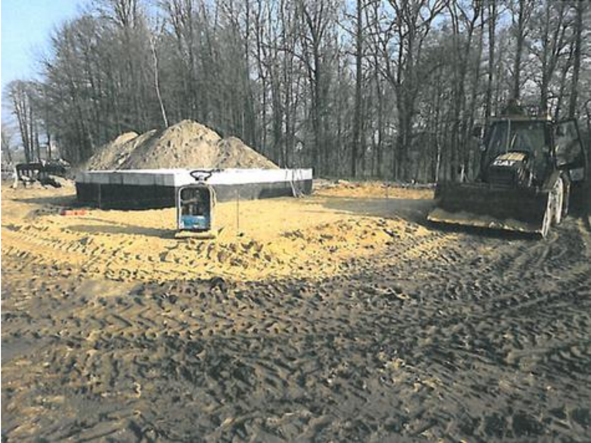
Photo No. 13. Reservoirs for filter beds.
