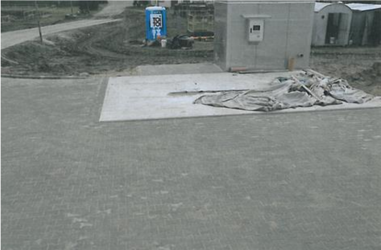
PhotoNo. 14. The catchment point for the sewage delivered.
