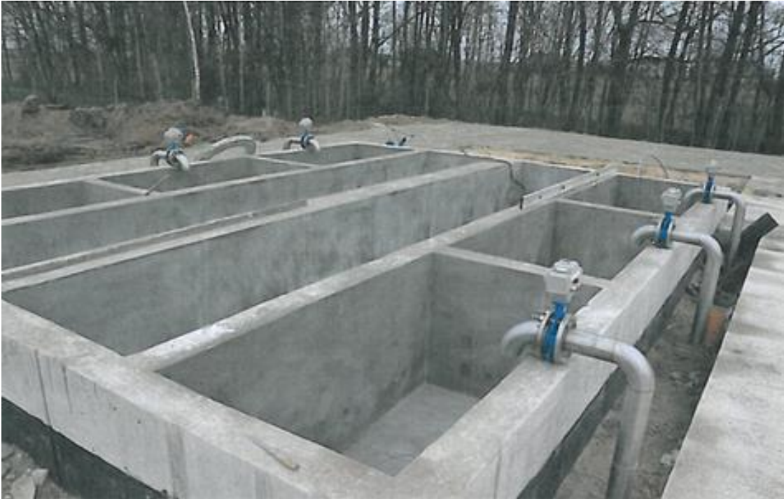
Photo No. 13. Reservoirs for filter beds.
