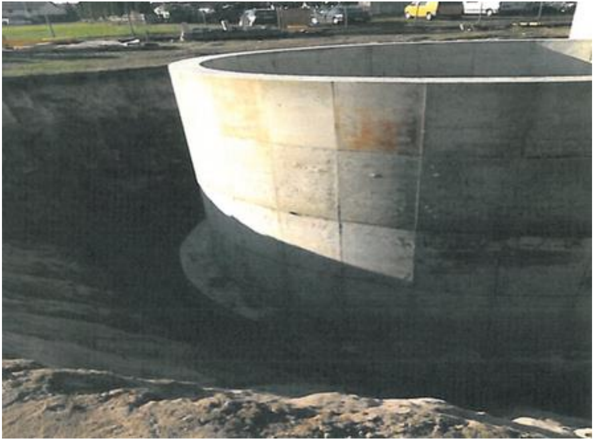
Photo No. 8. Installation of technology at the secondary settling tank.
