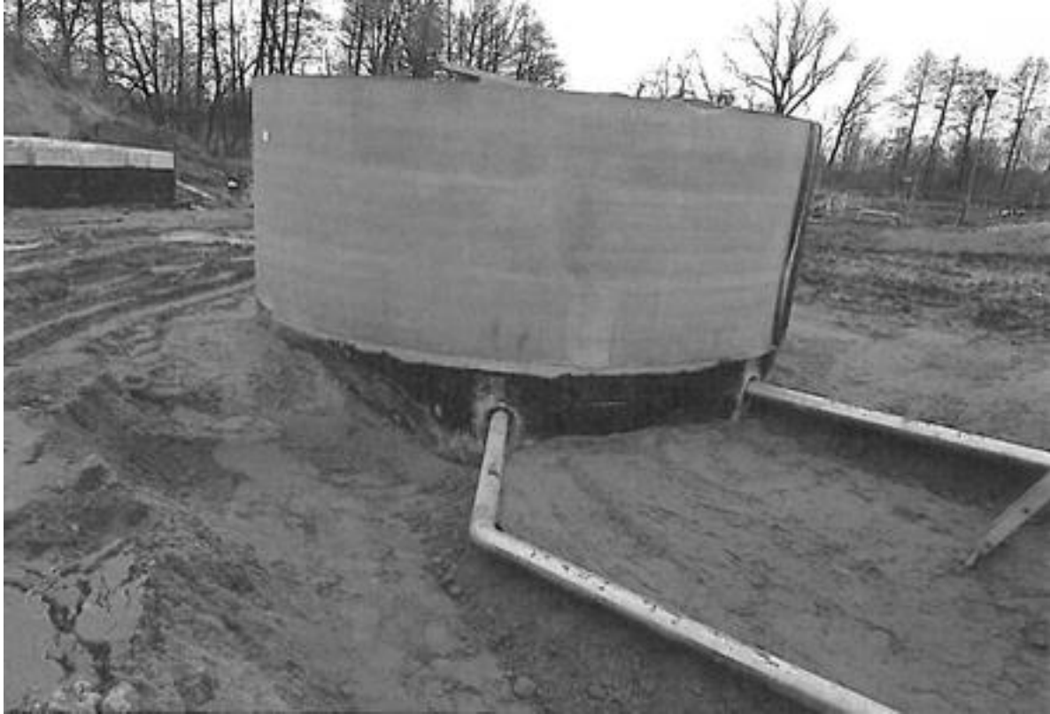
Photo No. 9. Installation of secondary settling tank technology.
