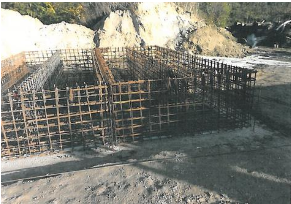
Photo No. 11. Reinforcement of filter bed tanks
