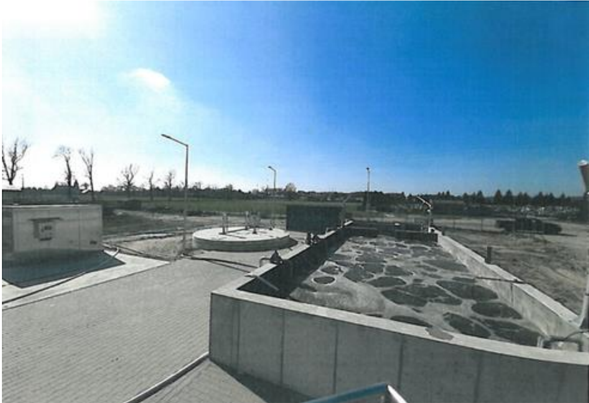
Photo No. 16. Technological start-up of industrial wastewater treatment plants.
