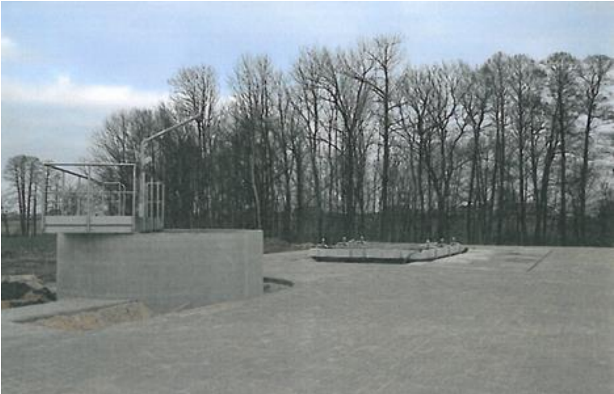
Photo. No. 15. Hardening the surface of the sewage treatment plant.
