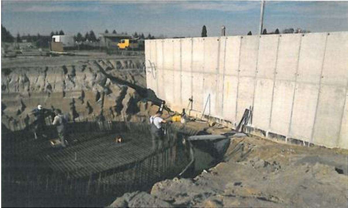
Photo No. 7. Walls of the averaging / surge tank.
