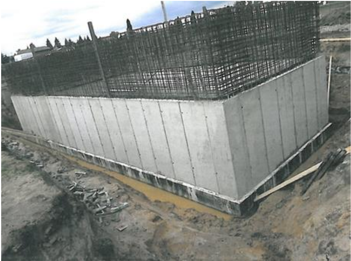
Photo No. 3. Performing internal insulation in the biological reactor.
